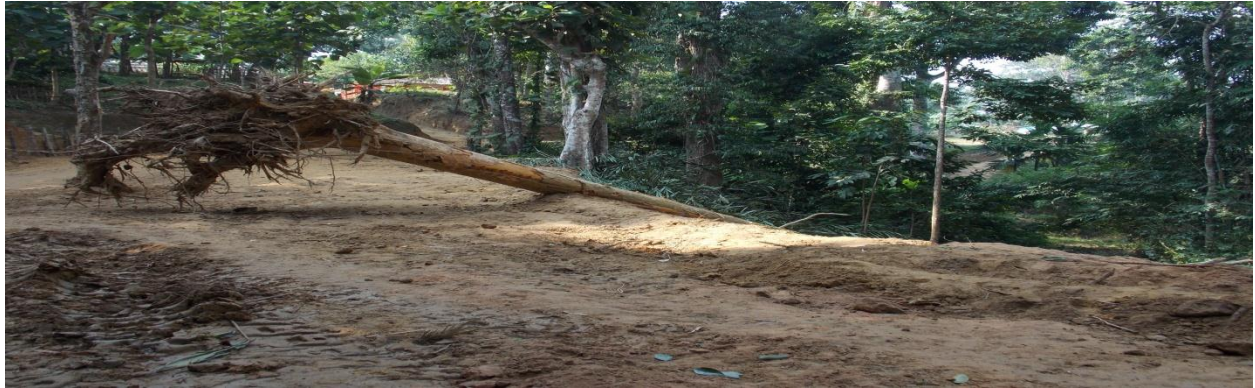
Village road widening
