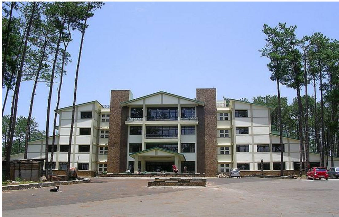
Figure 2: CENTRAL LIBRARY, NORTH EASTERN HILL UNIVERSITY.
