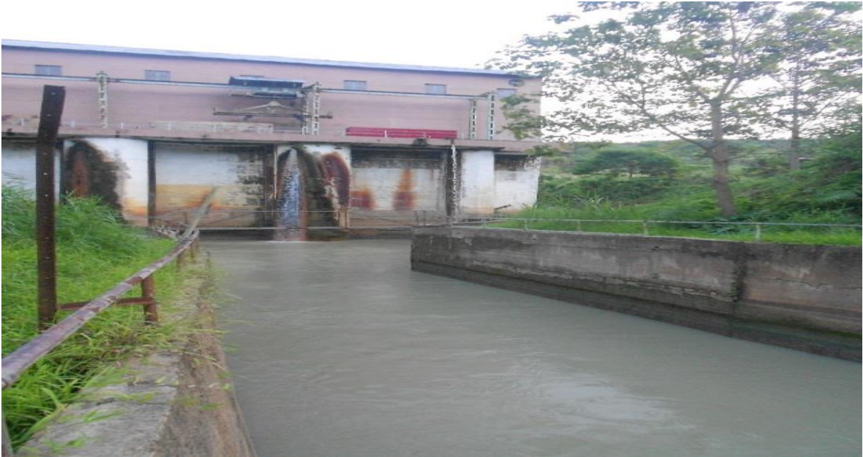
Photo plate 3.4: Power house outlet
