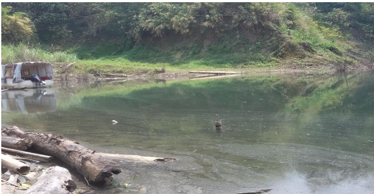
Photo plate 3.2: Site 2- Reservoir, where the flow of the water recedes with the development of the dam.
