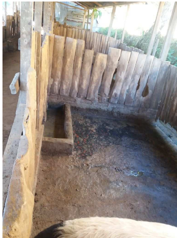
Fig. 3.1 Concrete Flooring of Pig Sty
