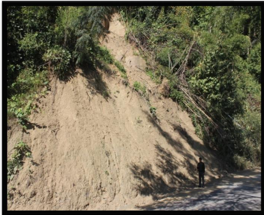
Fig. 3.4 : Collecting Landslide location points
