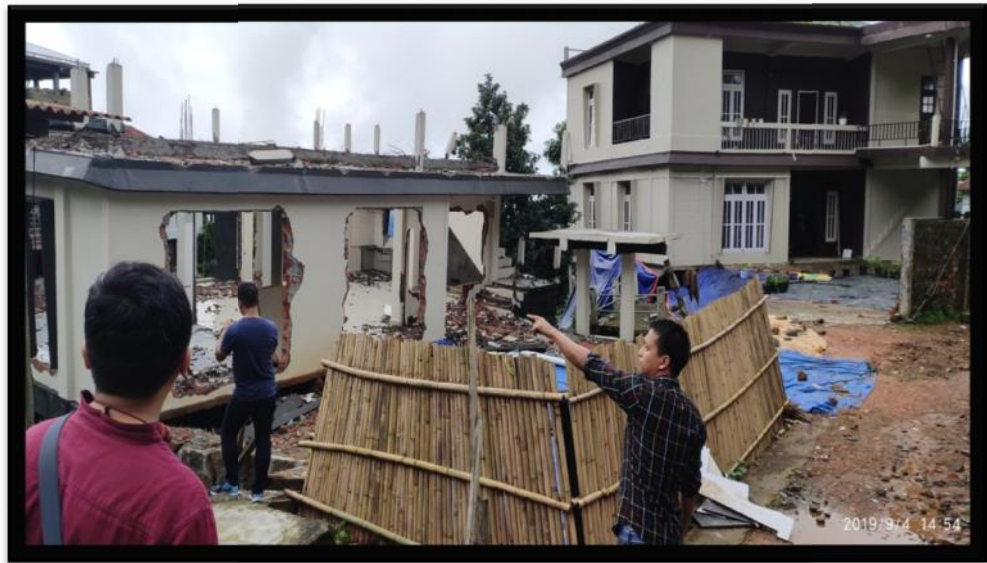
Fig. 3.7 : House destroyed by Landslide on 18 August 2019.
