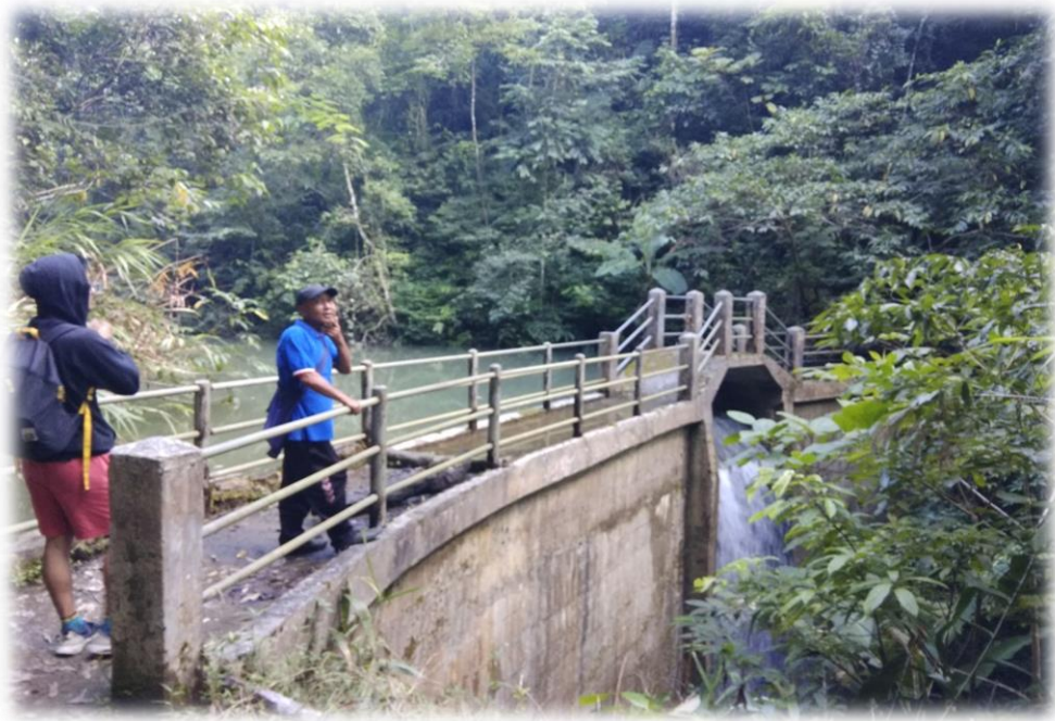
Plate C: Construction of a small dam by P.H.E at Lunglei District Park.
