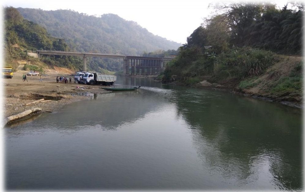
Plate B: Bridge construction at Bairabi
