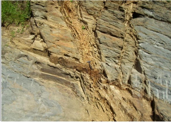
Plate 4.3 Development of Cracks on horizontal bed
