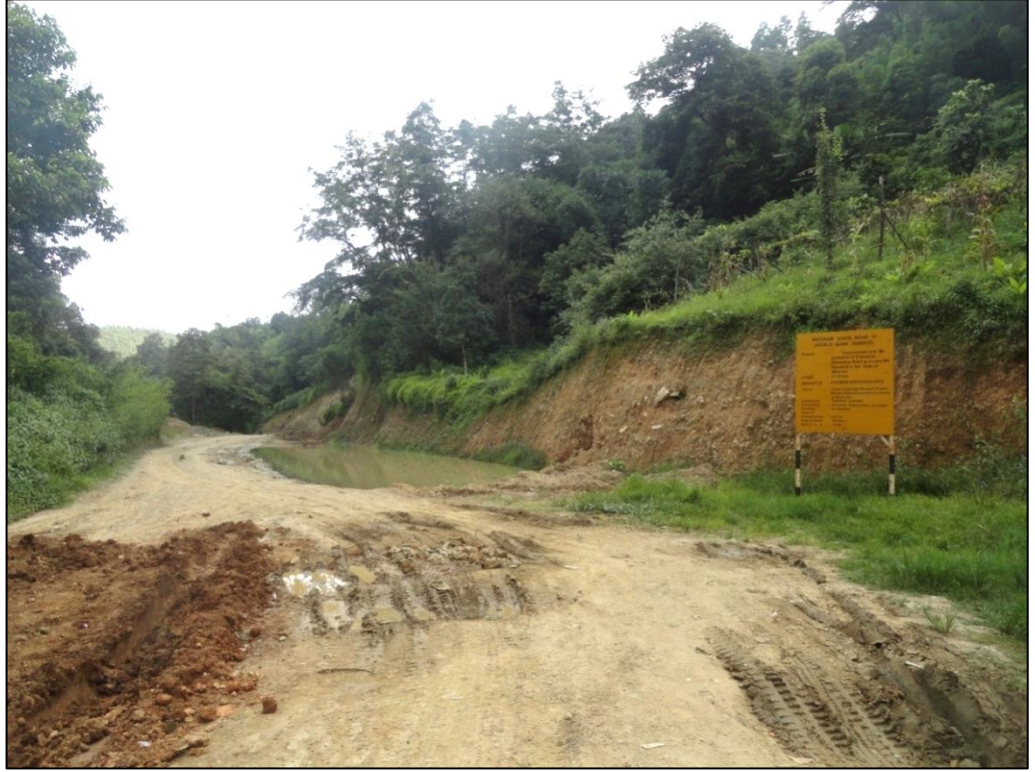
Photo 1: Champhai-Zokhawthar road project starting point at Champhai Police Check Gate.
