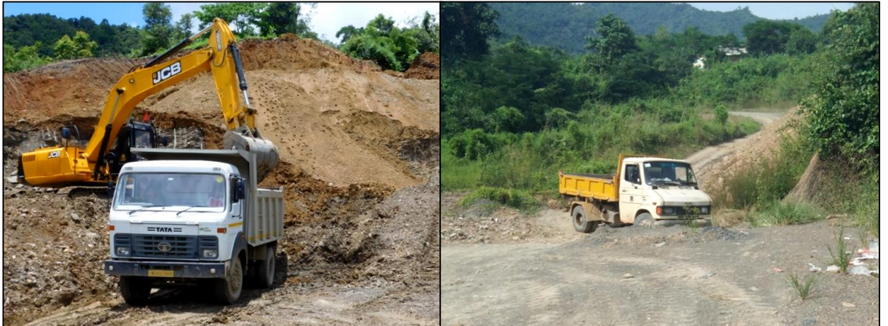
Photo 10: Excess soil is carried by trucks and deposited on Tiau river.
