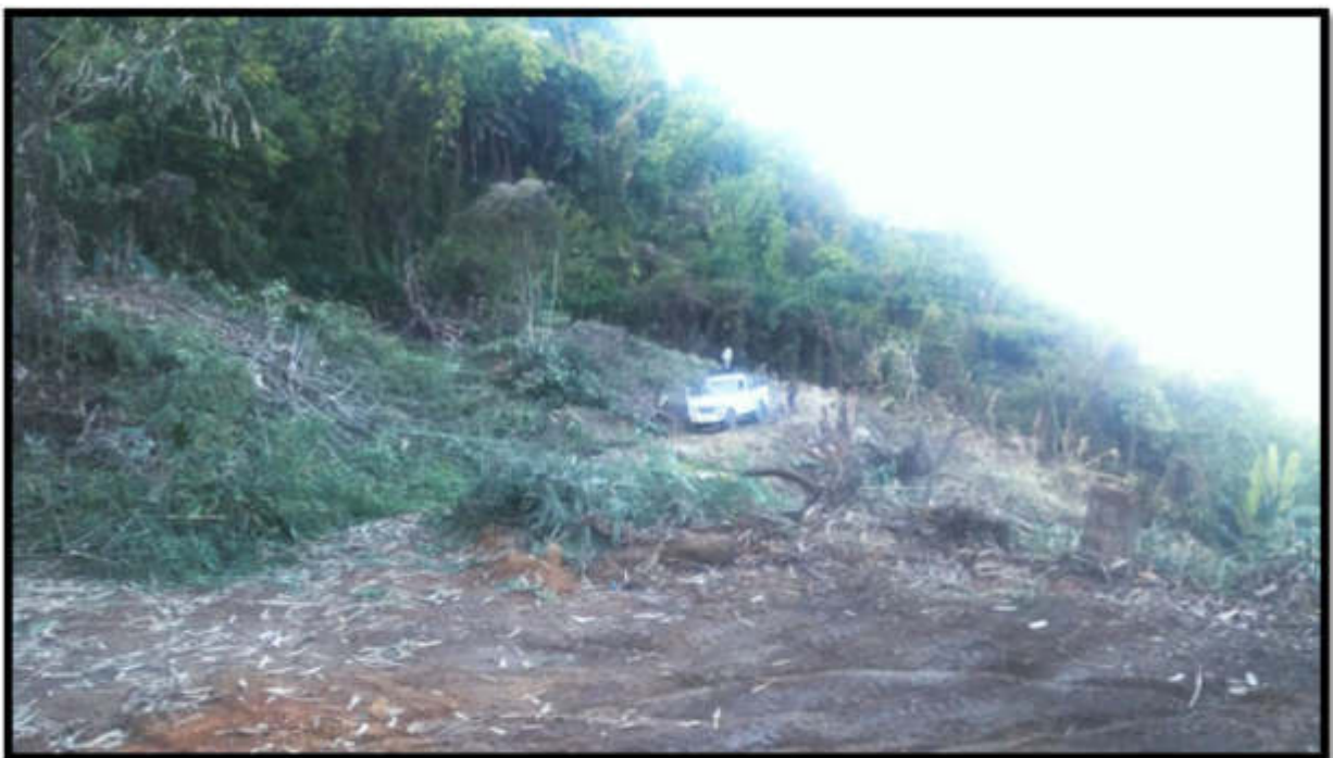
Photo B: Construction of link road for new farm land at Bualpui village.
