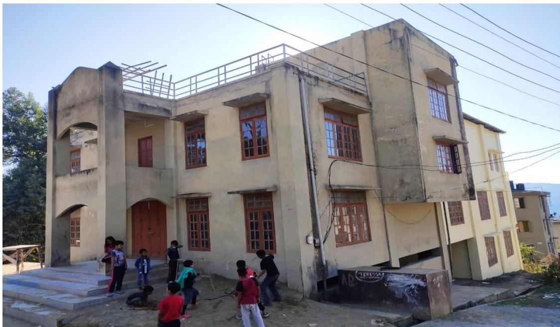
Photo plate No.11: The Community Centre at Lawipu. Source: Site visit
