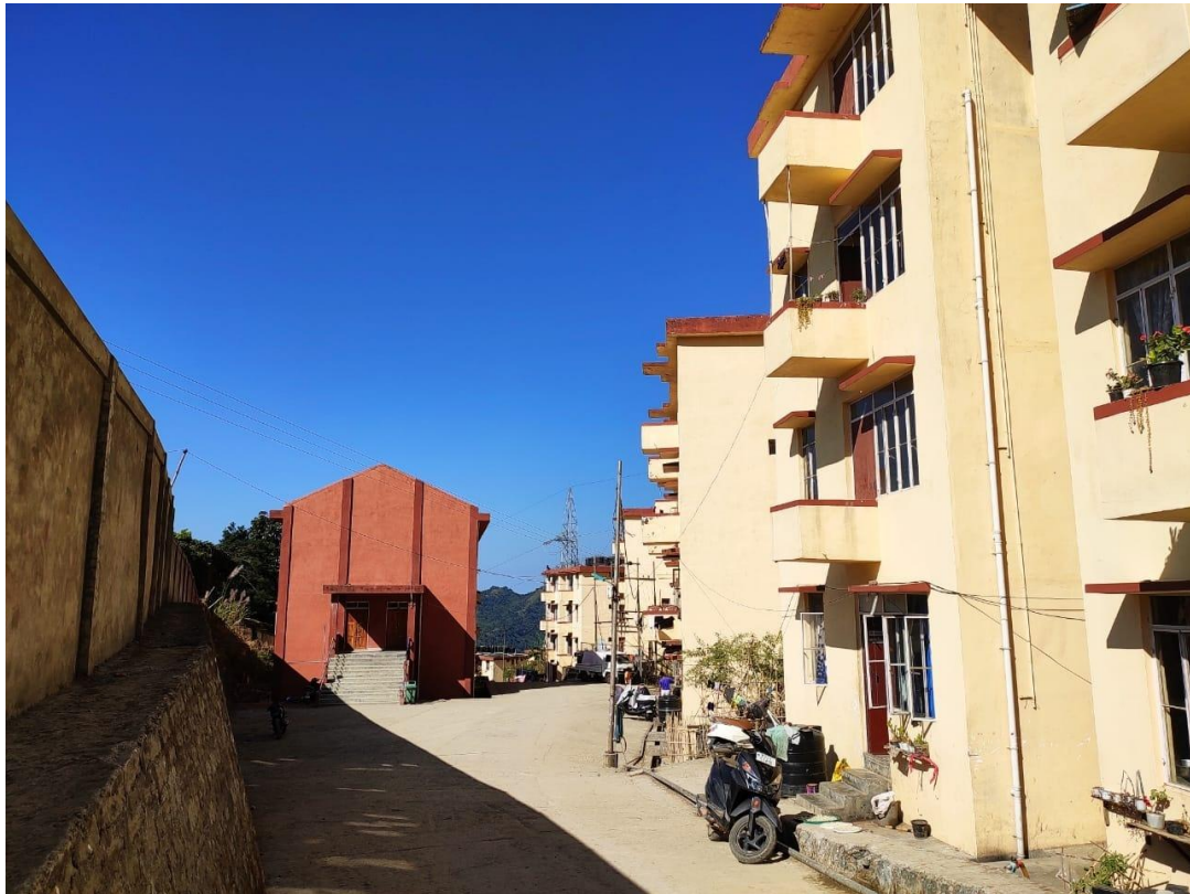
Photo plate No.6: BSUP Housing Complex, Edenthlar as on 2 nd January, 2021. Source: Site visit
