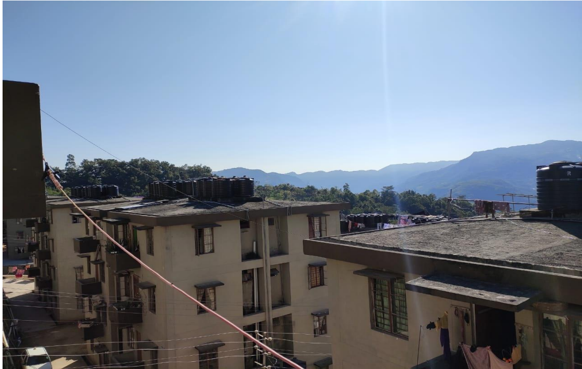
Photo plate No.2: EWS Housing Complex, Lawipu as on 2 nd January, 2021.
