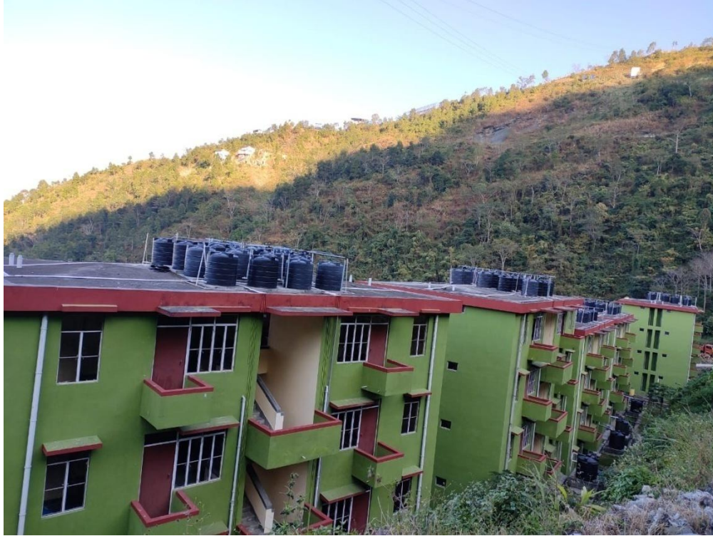
Photo plate No.15: Smaller water tanks at Durtlang.
