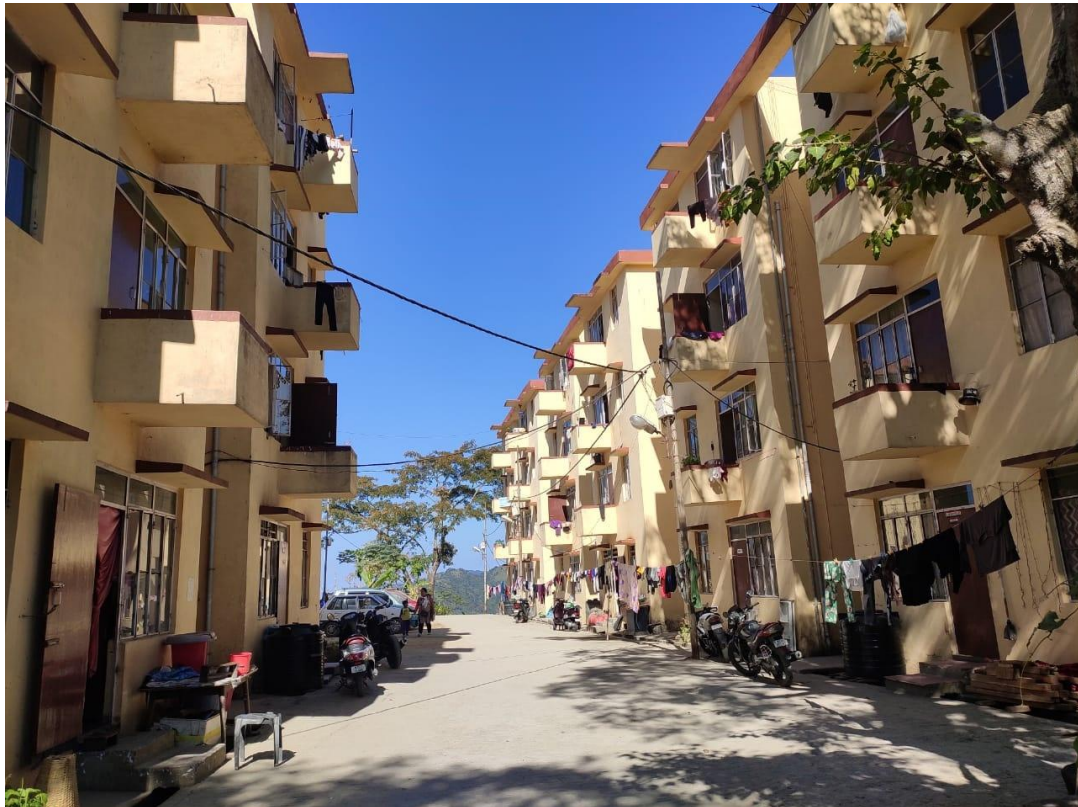
Photo plate No.5: BSUP Housing Complex, Rangvamual as on 2 nd January, 2021. Source: Site visit
