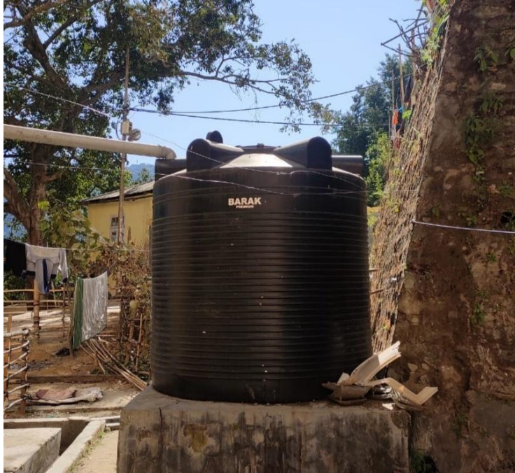
Photo plate No.13: Large water tank at Edenthar. Source: Site visit
