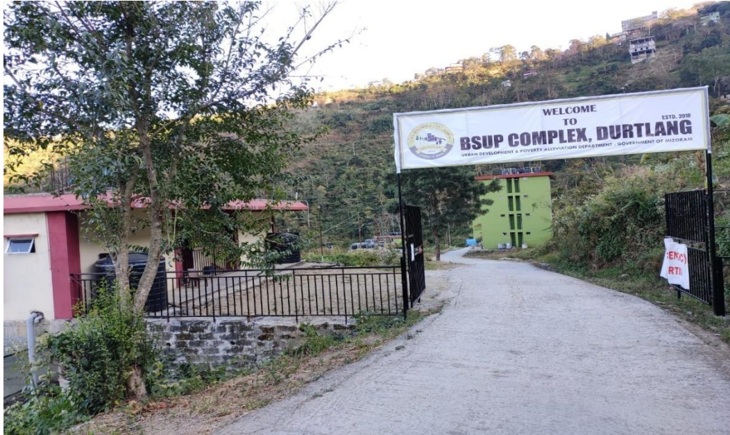
Photo plate No.3: BSUP Housing Complex, Durtlang as on 2 nd January, 2021. Source: Site visit
