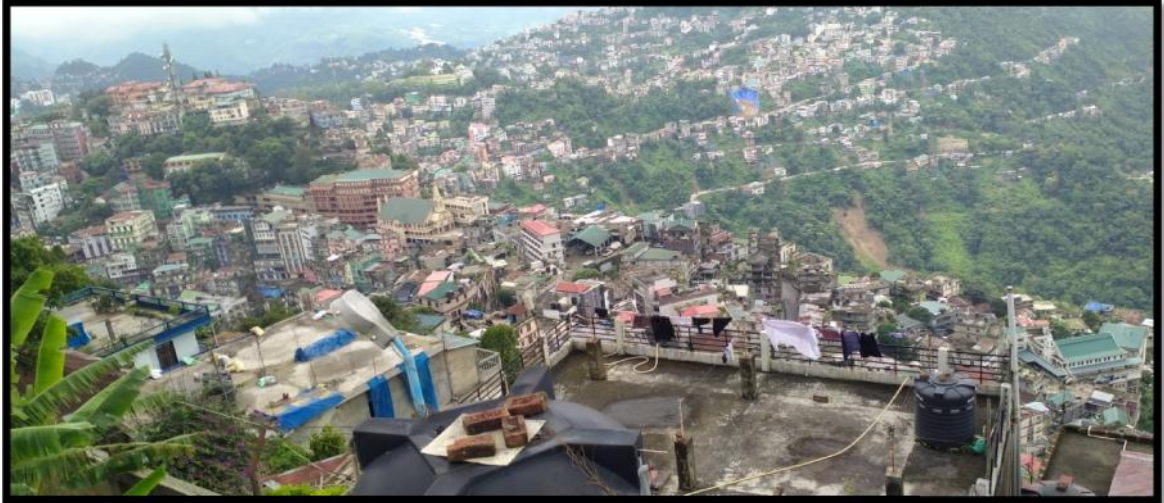
Types of roof in some parts of western slope of Aizawl city ridge
