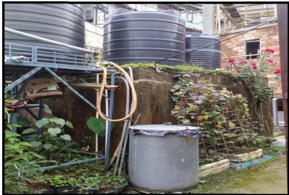
RCC water tank, constructed on the ground in Ramhlun locality.
