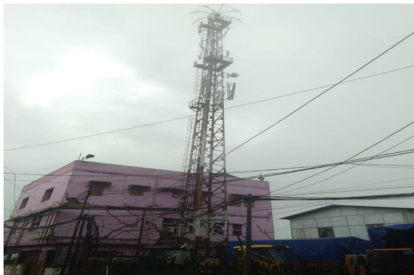
Fig. 4.6.1: Tower at Lunglei Bazar Veng (BSNL).
