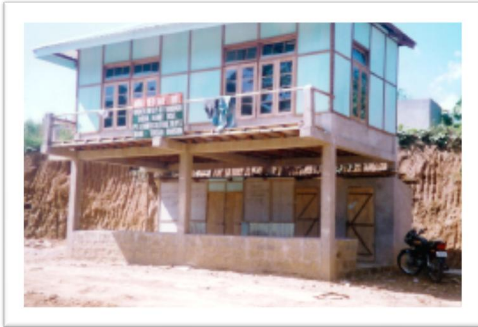
Exhibit 2.14 A rural haat in Mamit constructed by the Government
