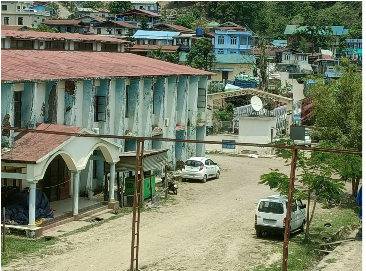
Fig.3.1 Land Custom Station Building at Zokhawthar (India – Myanmar border)
