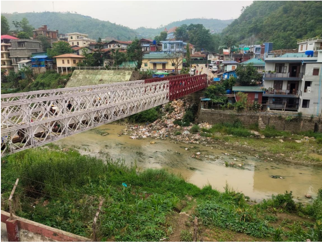
Fig 4.8 River Tiau at India and Myanmar Boundary during dry season
