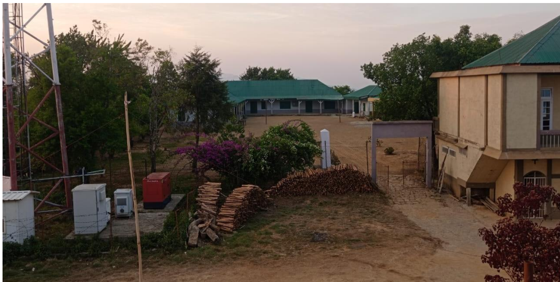
Fig 4.3 High School at Thingsai
