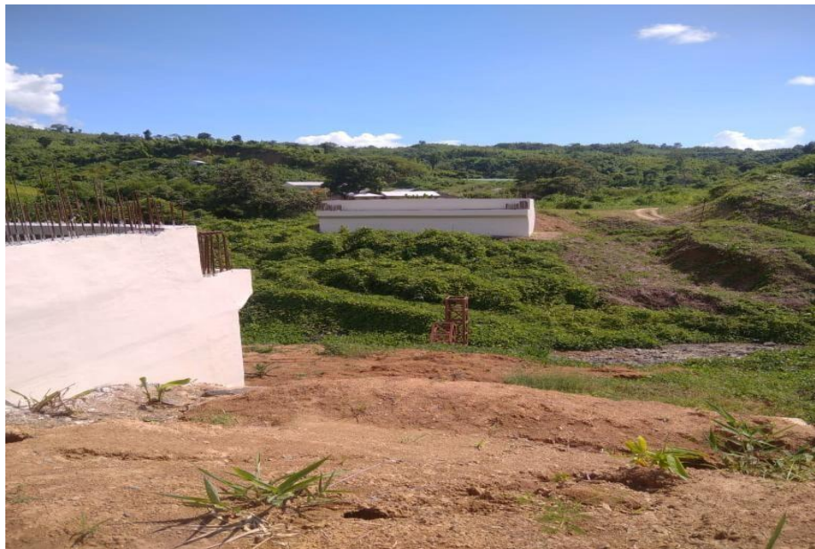
Fig. 4.11 A under-construction bridge to connect India – Myanmar at Zochachhuah.
