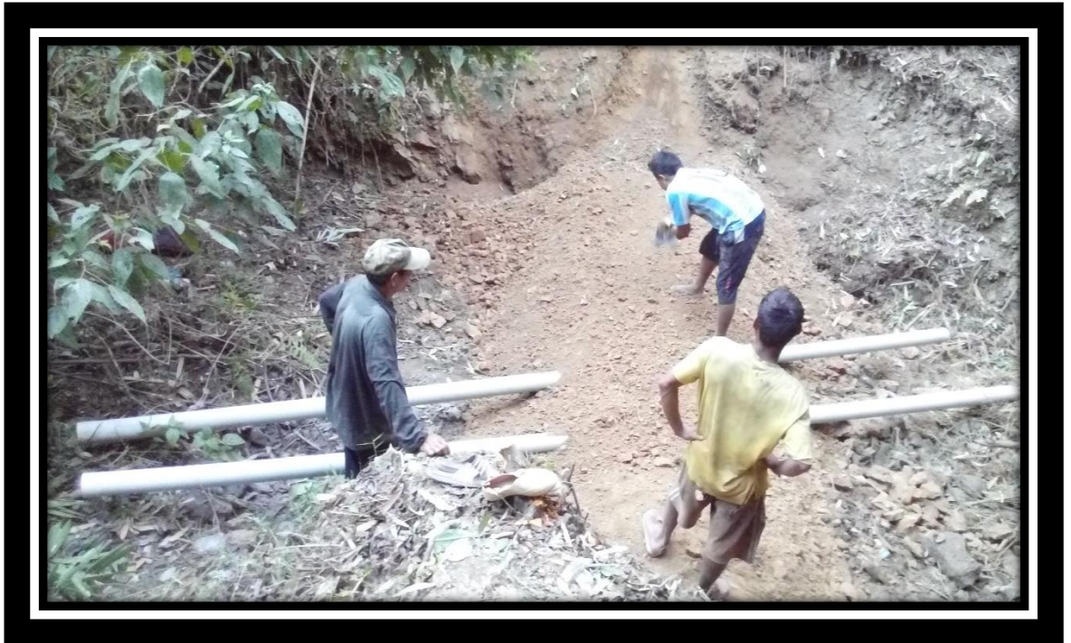
Plate 19 Daily workers of Bru constructing fish pond
