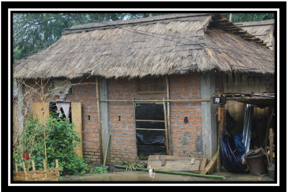
Plate 4 RCC under construction
