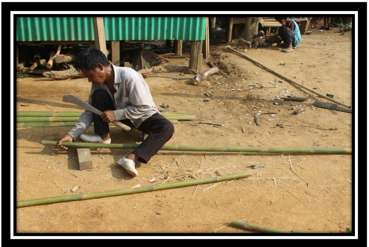
Plate 18 Bru man making dap for construction of house
