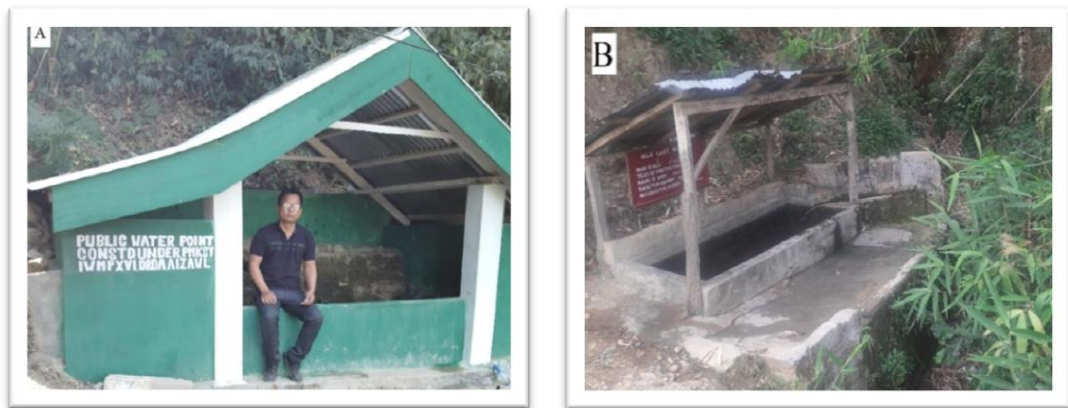
Plate 6.2: A) Spring shed under PMKSY, Hmuifang. B) Spring shed under LAD, Thingsulthliah. Source: Author
