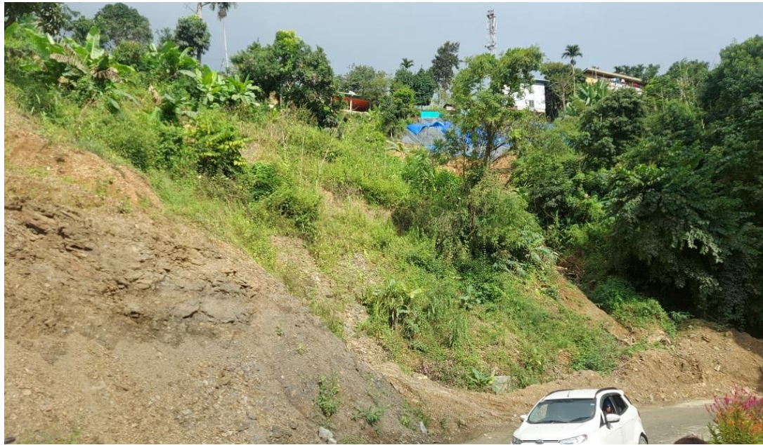
Location 7. Landslide (Translational type) near National highway, Hualngo.
