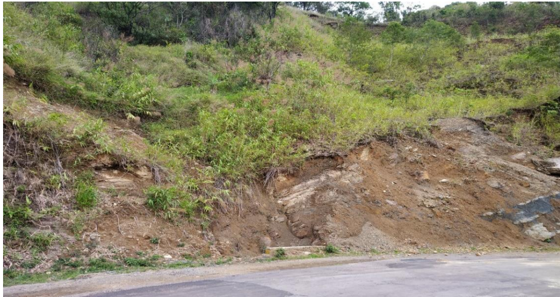
Landslide location 1. Landslide (Translational type), Chamring.
