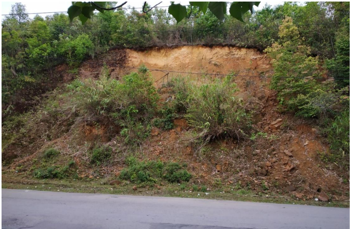
Location 2. Landslide (Translational type), Maubuang
