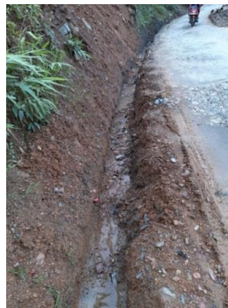
Fig. 4.10 Emanation of groundwater from the hill slope
