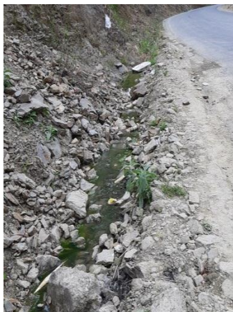
Fig. 4.10 Emanation of groundwater from the hill slope
