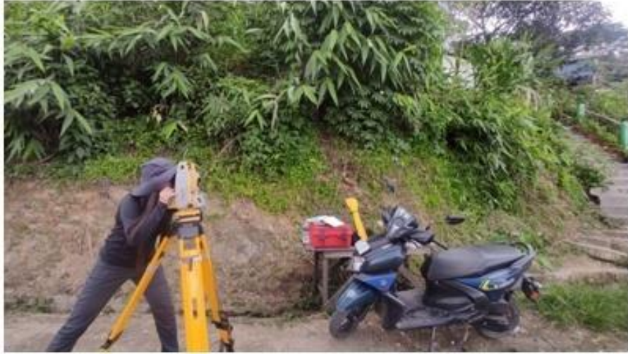
Figure: Total station survey
