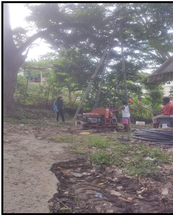
Figure 4.13: Core Drilling at Location-2
