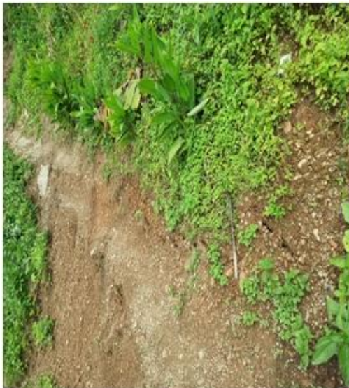
Figure: Crown of landslide
