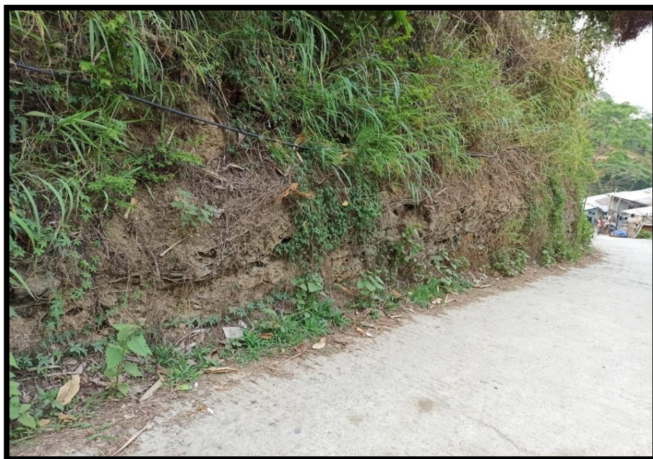
Figure 5.3. Gabion wall constructed in the road section of the middle area
