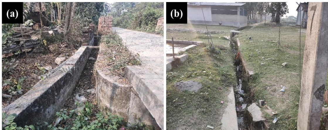
Figure 8.8: Difficulties in wastewater drainage facilities (a) nonfunctional wastewater drainage systems in Abua village, and (b) broken wastewater drainage facilities in Srinagar village; Source: By author
