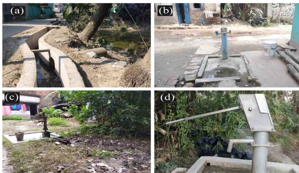
Figure 6.4: Drainage infrastructure in the study villages (a) open drainage facilities in Abua village, (b) closed drainage facilities in Sontoshpur village, (c) a household has no drainage facilities in Kamra village, and (d) no drainage facilities in Narayanganj village; Source: By author
