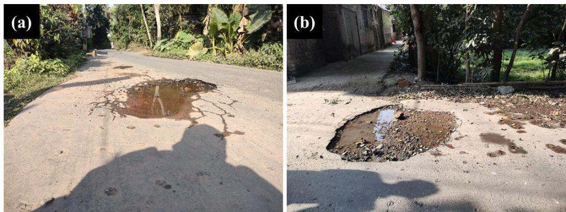
Figure 8.1: Effect of water pipe leaks in Sontoshpur village (a) water pipe leaks impact community access in Sontoshpur village, and (b) deteriorating road ambient due to persistent leaks; Source: By author
