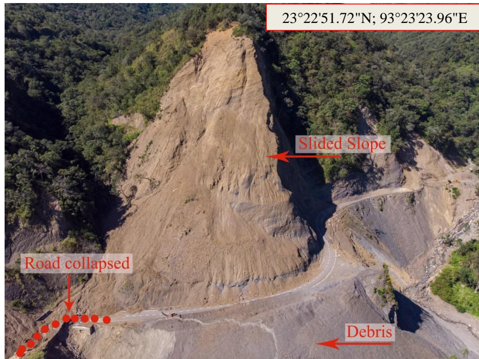
Fig. 4.3 Road and retaining wall collapsed
