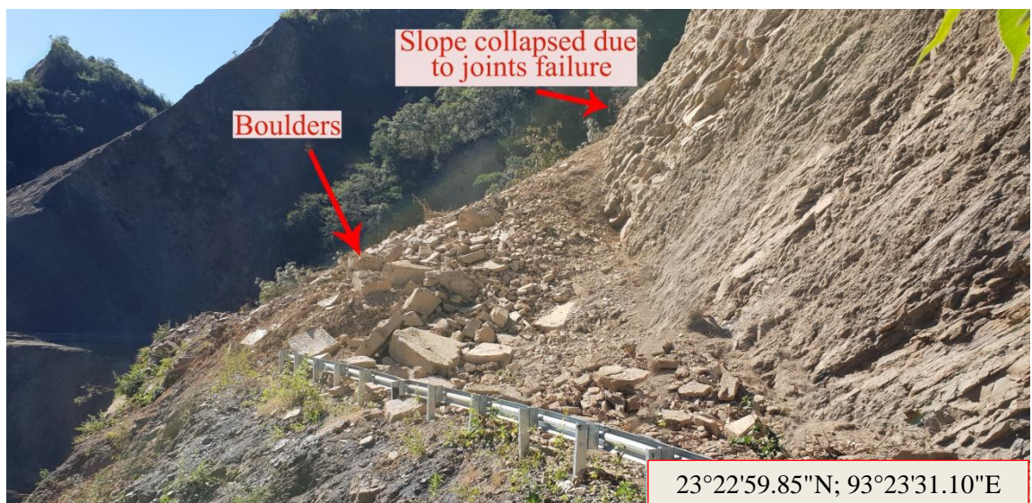
Fig. 4.4 Slope Failure ( The slope collapsed due to the failure of the joints. Boulders that fell from the slope completely blocked the road )
