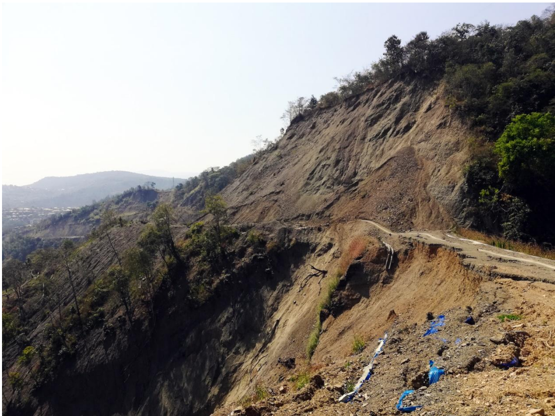
Fig. 7 Retaining wall collapsed due to slope failure
