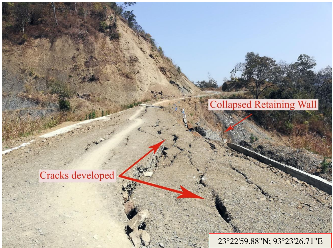
Fig. 4.5 Collapsed Retaining Wall ( Due to the collapse of the retaining wall, cracks developed on the road )
