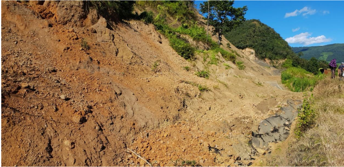
Fig. 3 Landslide debris completely blocked the road
