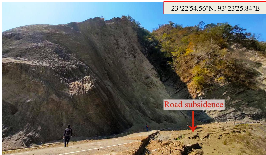
Fig. 4.6 Bedding Plane Failure
