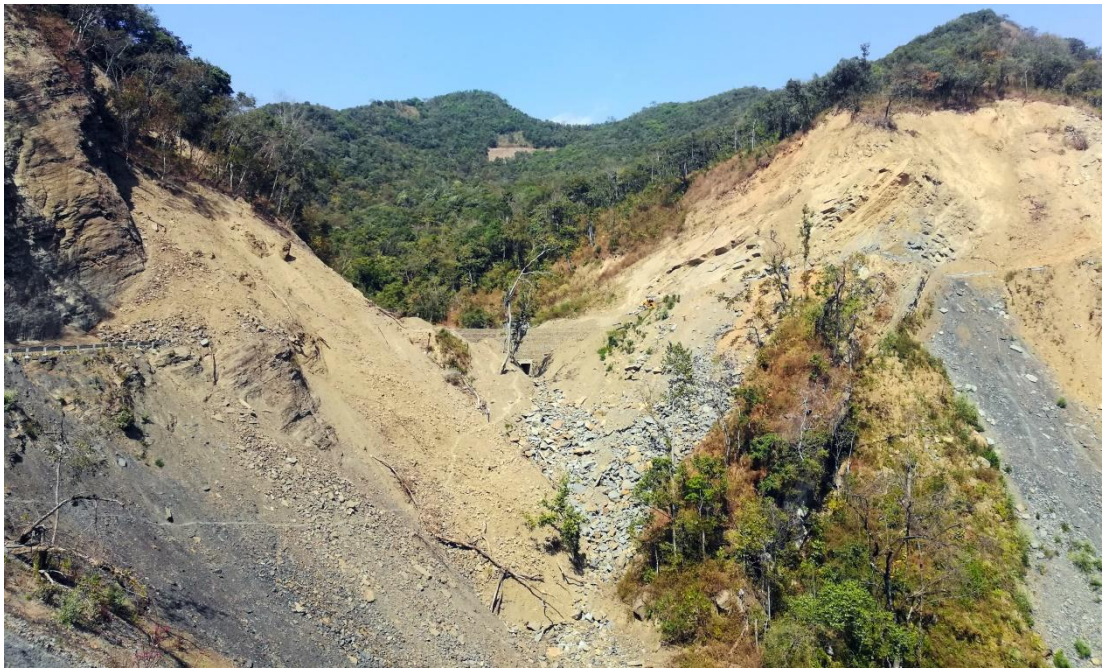
Fig. 6 Collapsed Road and slope
