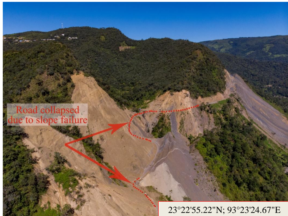
Fig. 4.1 Collapsed Road and Landslides ( The road collapsed and was inaccessible due to landslide. Dotted lines represent the road which was collapsed )
