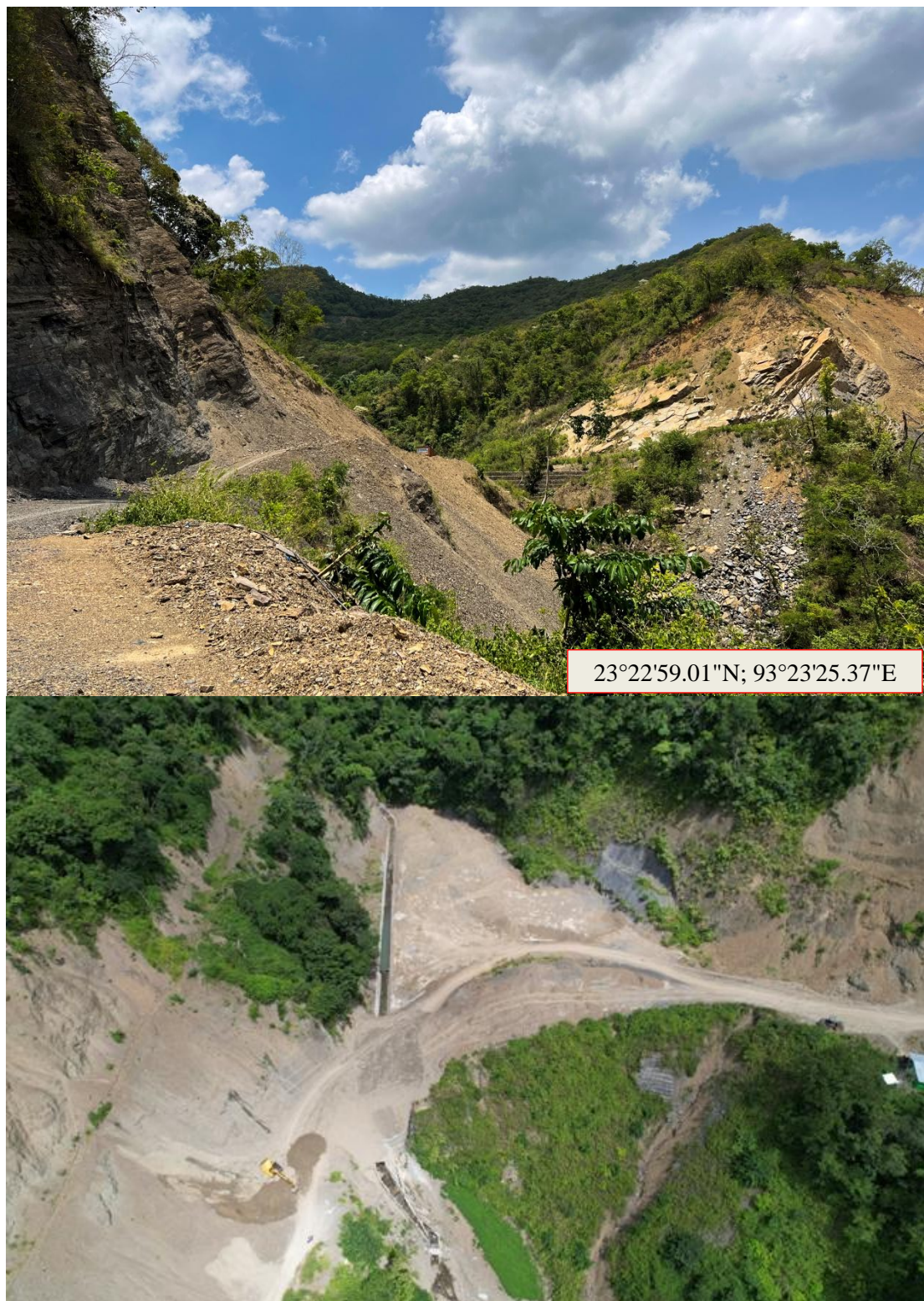
Fig. 4.36 Field photograph of failed slope in LS3
