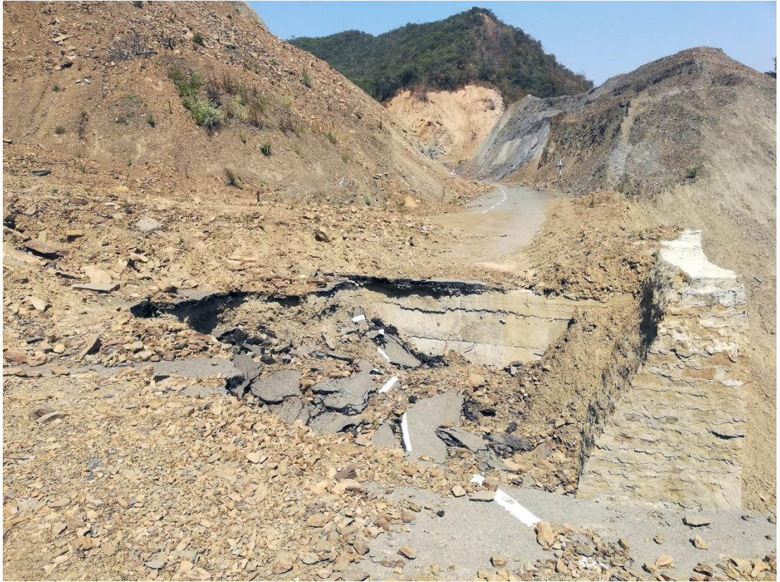
Fig. 8 Road, Curvert and Retaining collapsed
