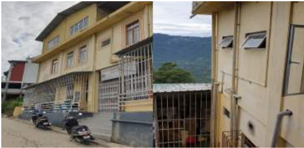
Figure 5.8: Building structure of UPHC Chawlhmun
