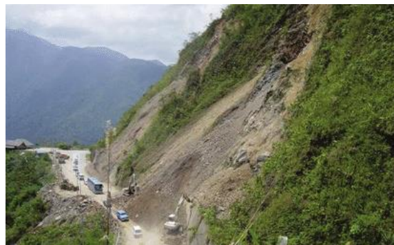
Fig. 1.2(b): Images showing man-made slope. (nativevegetation.org)
