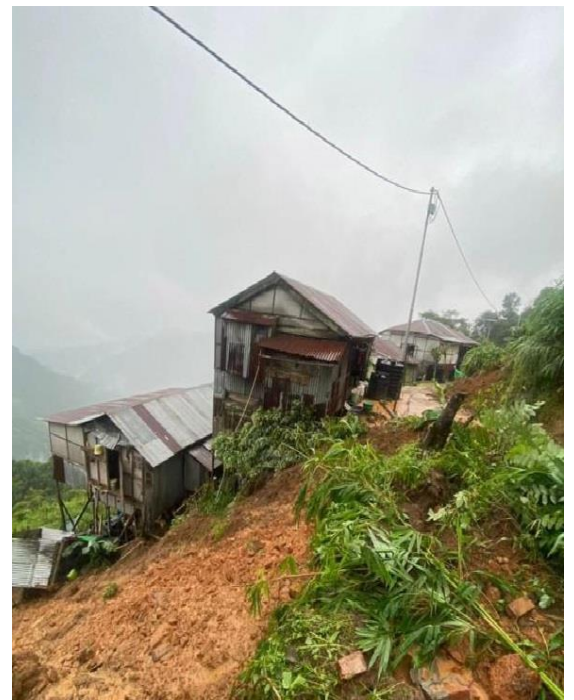
Fig.1.1: Images showing slope failure due to construction activities in Aizawl city.
