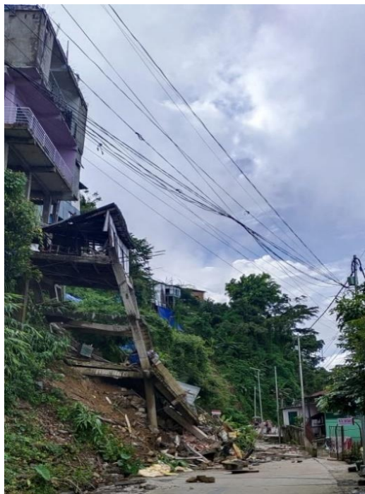
Fig.1.1: Images showing slope failure due to construction activities in Aizawl city.
