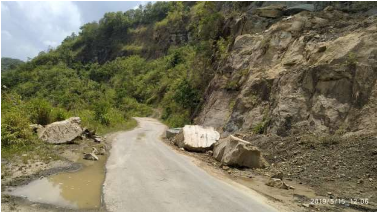
Location 4.Landslide (Rockfall), Tlungvel Quarry.
