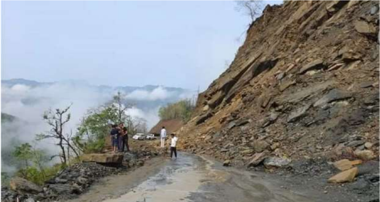
Location 7.Landslide (Rockfall), Keifang Quarry.
