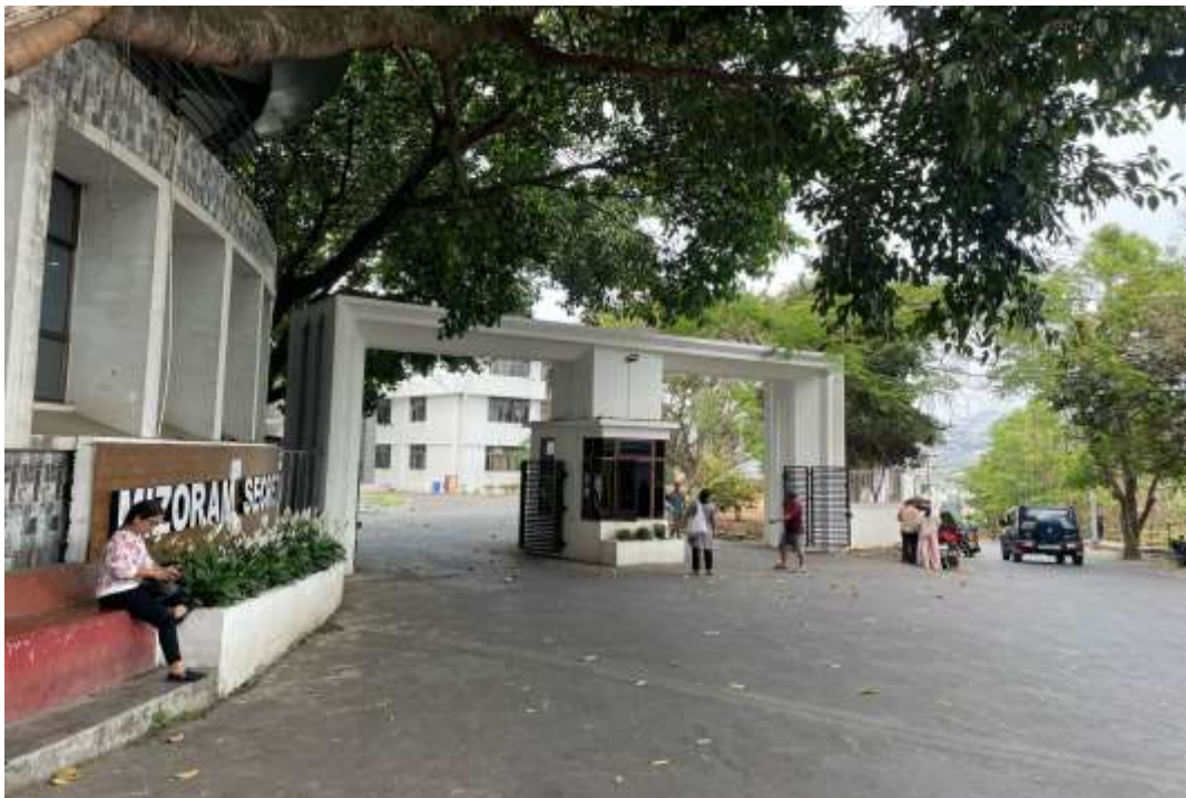
RS-CO11 (New capital complex, Mineco)
