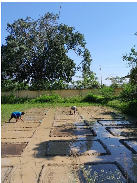
Plate 9: Preparation of levees
