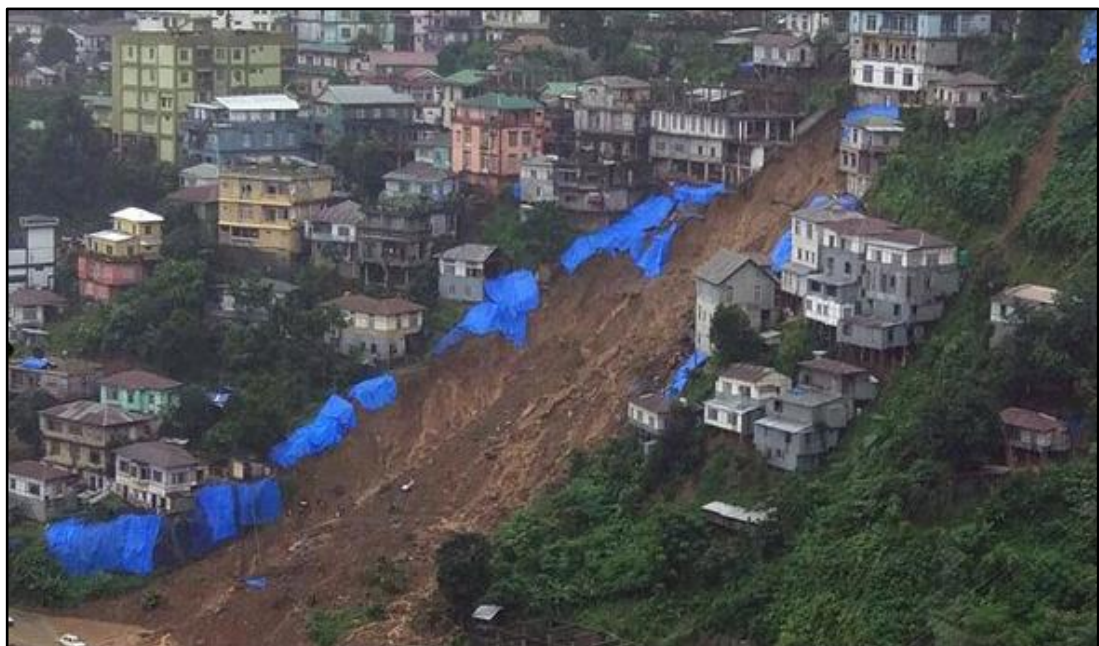
Photo Plate 3.12 Recurrent landslide activity at Hunthar Veng
