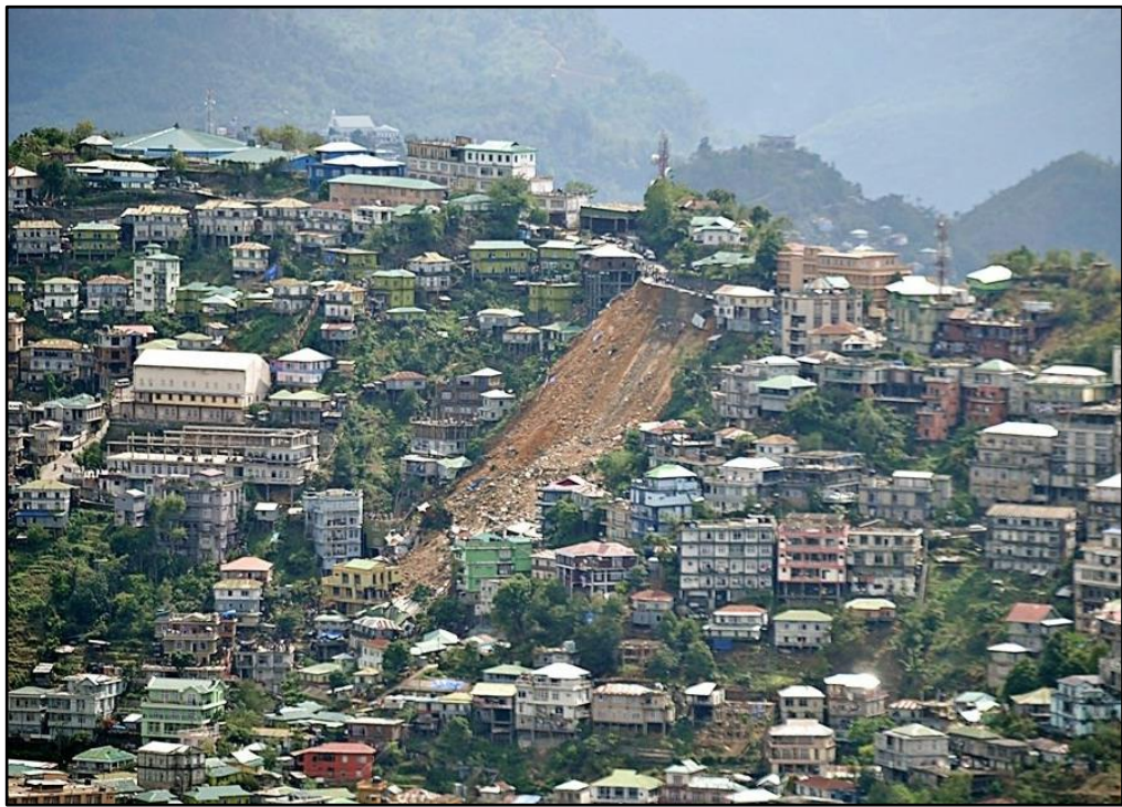
Photo Plate 3.8 The Laipuitlang landslide (11 May, 2013) was one of the deadliest incidents
