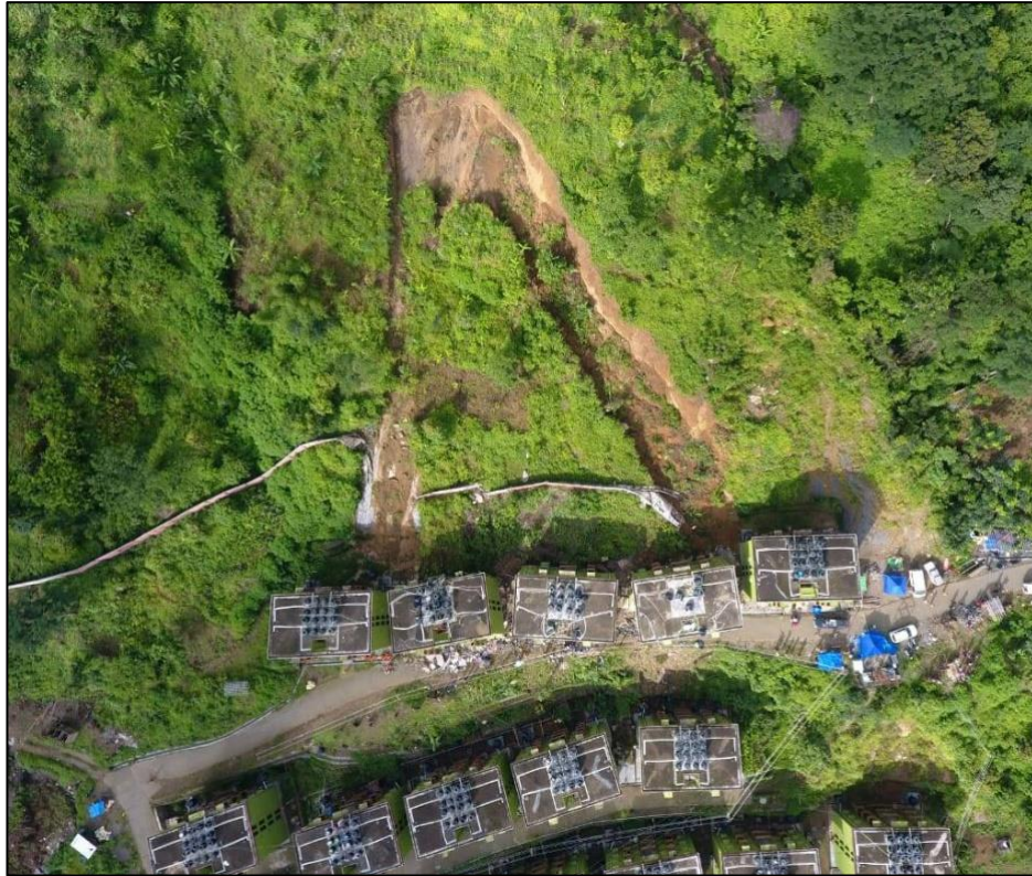
Photo Plate 3.10 The landslide at the BSUP complex, Durtlang (2 July, 2019)
