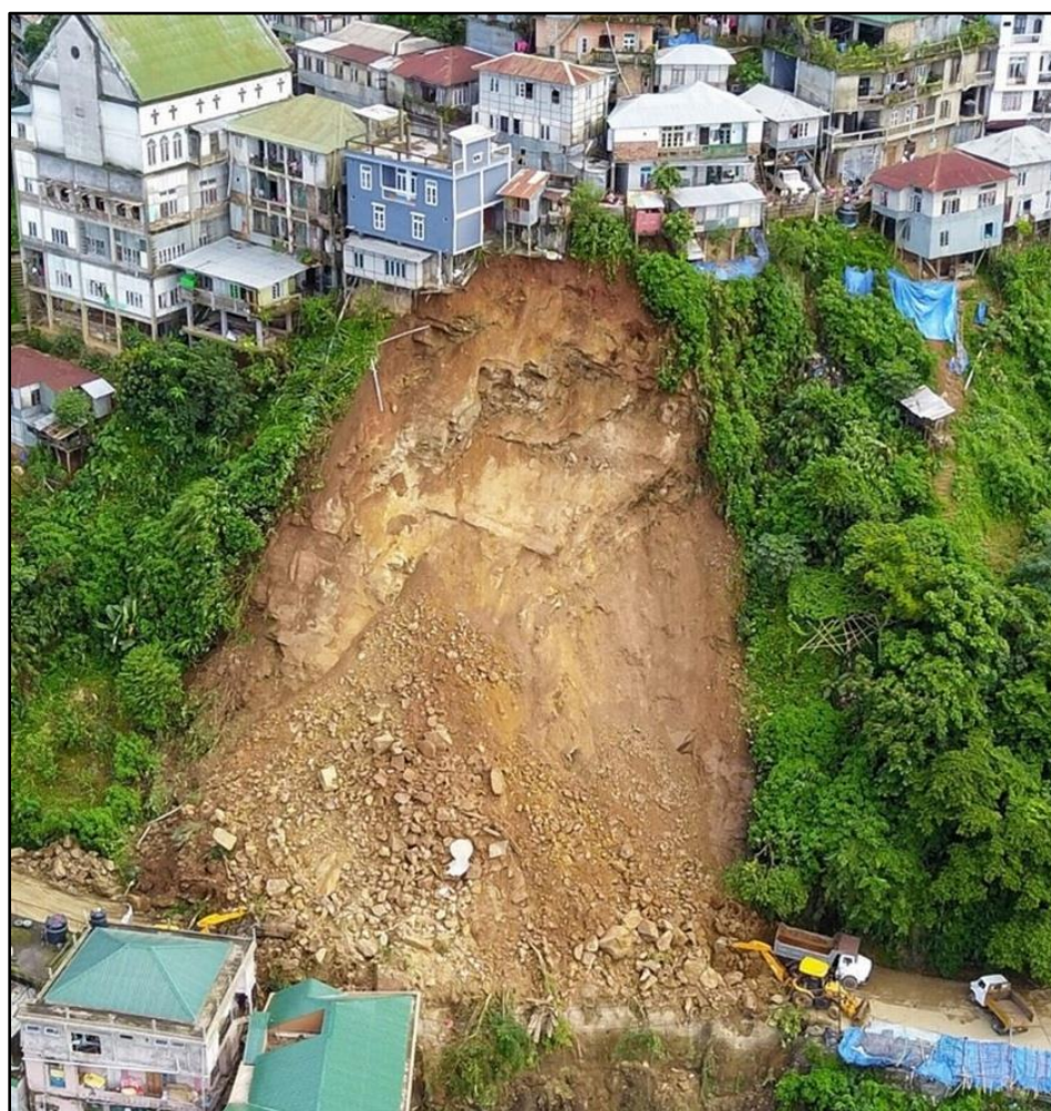
Photo Plate 3.9 The landslide along Bawngkawn-Thuampui road corridor (26 July, 2019)
