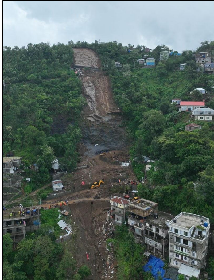
Photo Plate 3.11 The landslide at Melthum (28 May, 2024)
