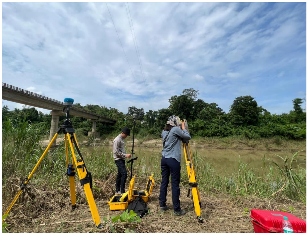
Figure 8.6 River line survey during monsoon at Bairabi using Total Station
