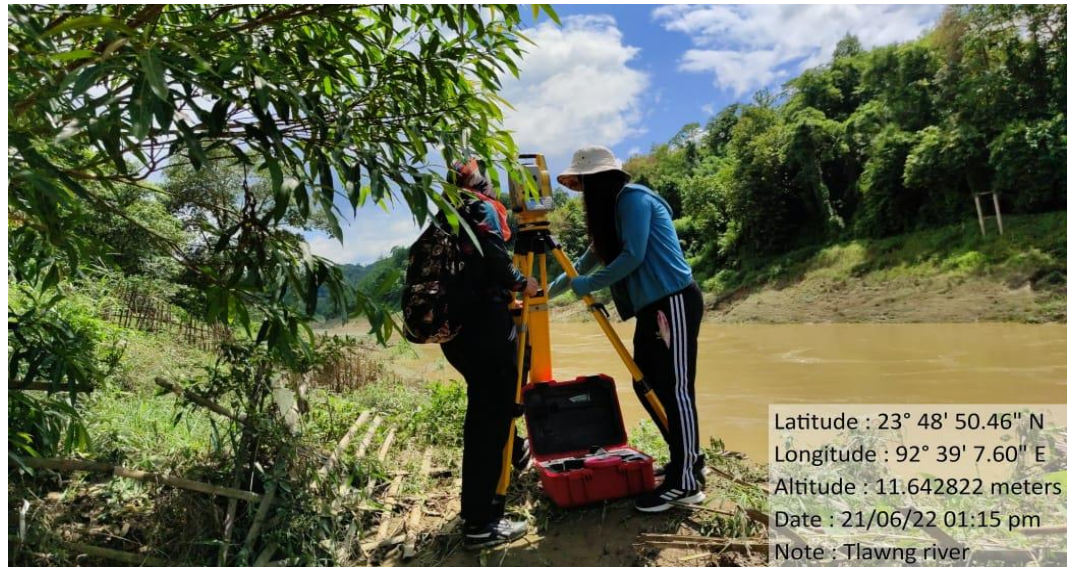
Figure 8.5 River line survey during monsoon at Sairang using Total Station
