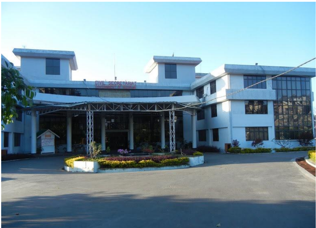
Photo Plate 3.12: Zone 4- Civil Secretariat Complex, Khatla
