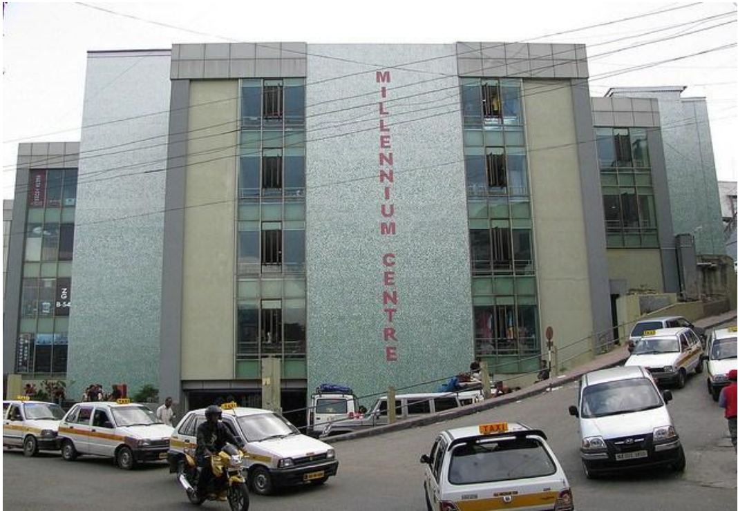
Photo Plate 3.5: Zone 2- Millennium Centre, Dawrpui
