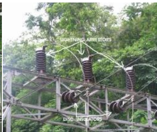
Lightning Arrester at Pump House No-I
