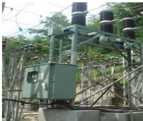
Vacuum Circuit Breaker at Pump House No-I
