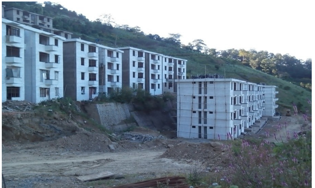
EWS Housing, Durtlang (As on 30 th October, 2015)
