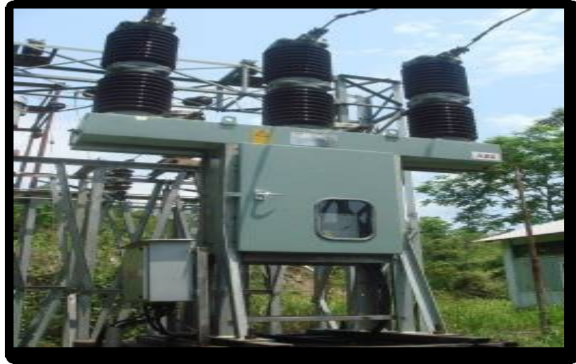
Vacuum Circuit Breaker at Pump House No-II
