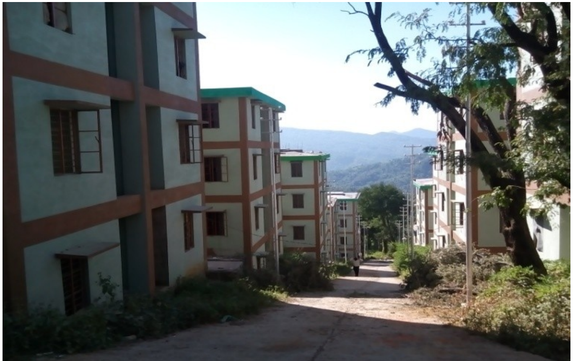
EWS Housing, Lawipu (As on 29 th October 2015)
