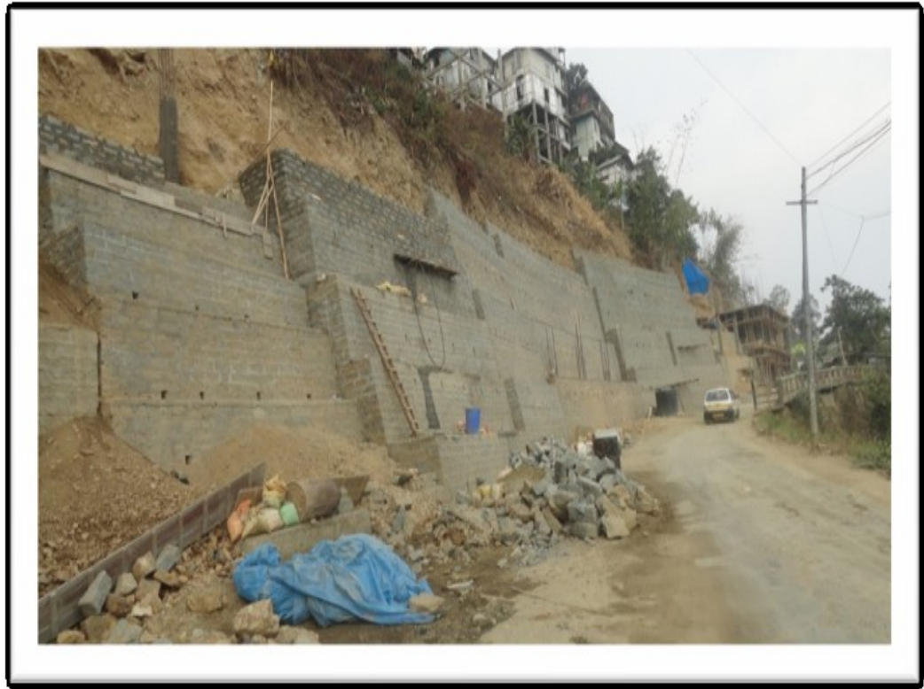
Widening of Mizoram University road in progress (As on 6 th April, 2013)
