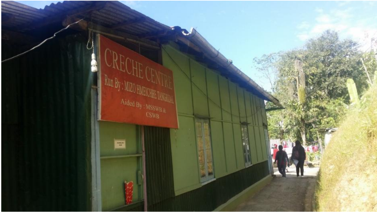
The MHIP Headquarter, Khatla Crèche Centre as on 1/12/2016
