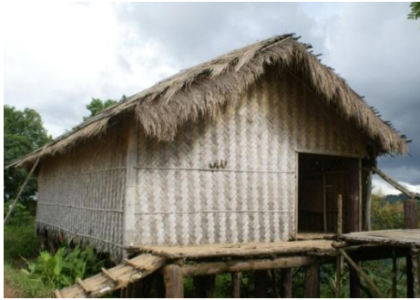
Fig: A typical Mizo house (Front view) Fig: A typical Mizo house (Side view)
