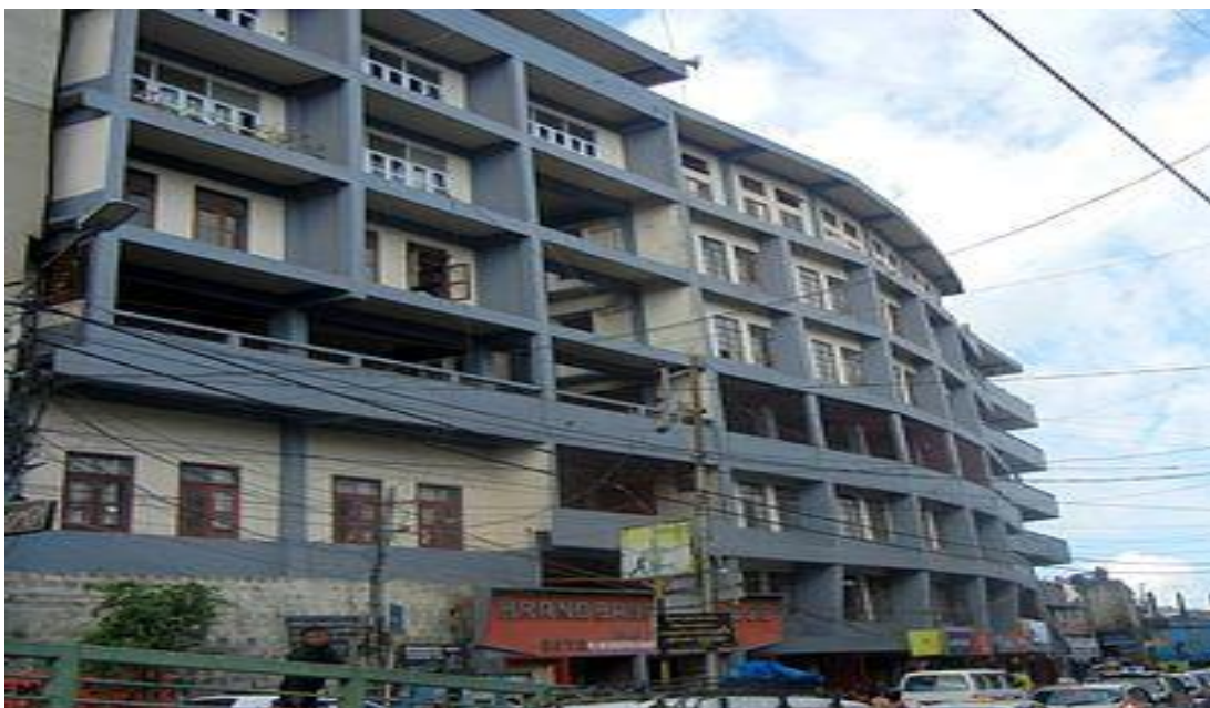
Figure- 3.5: Government Hrangbana College Building
