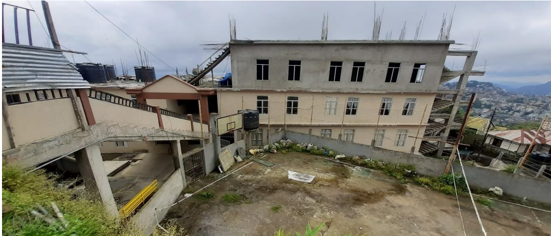
Figure- 3.17: Government Johnson College Building
