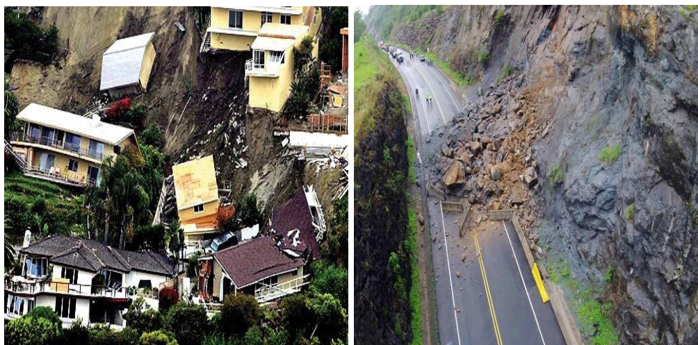
Figure- 2.9: Landslide disaster
