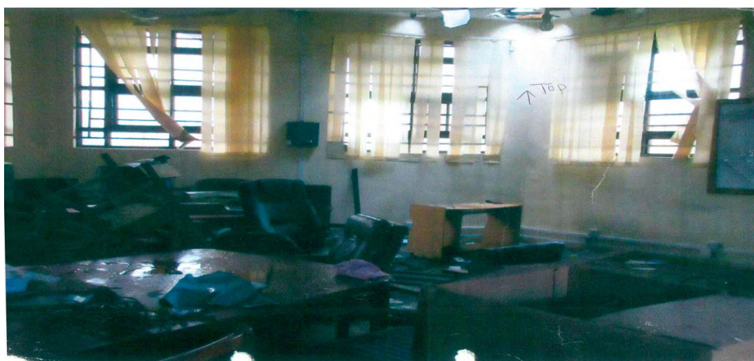
Figure- 2.15: Technical room of the Computer Resource Centre at the University Library, FUTA after the fire in 2014 (Source: Google Image)***
