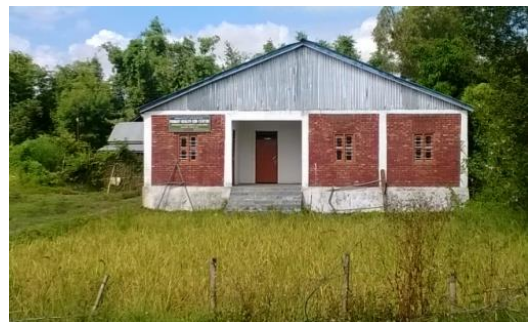
Photo 5 Chairel Sub-Centre (health center)
