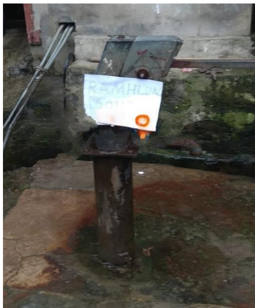
Photo plate 3.3: Site 3- Ramhlun South Handpump (Near Ramhlun South Presbyterian Church)
